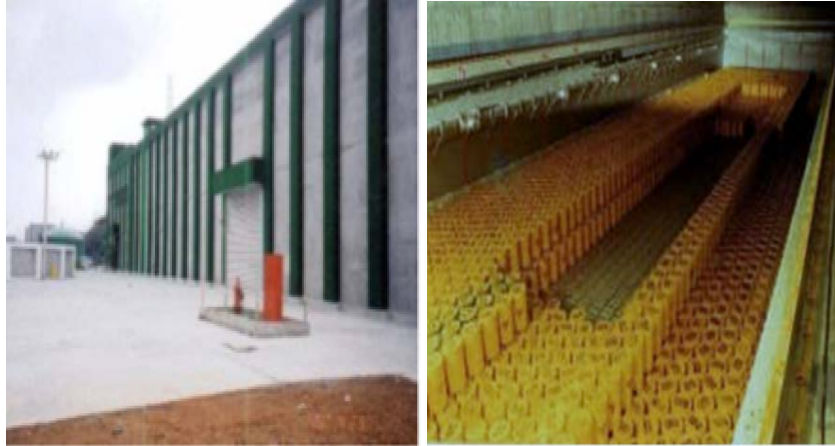
Fig. 2: Left, Building of a Taipower Indoor LLW Storage Facility; Right, Inside of a Taipower Indoor LLW Storage Facility
